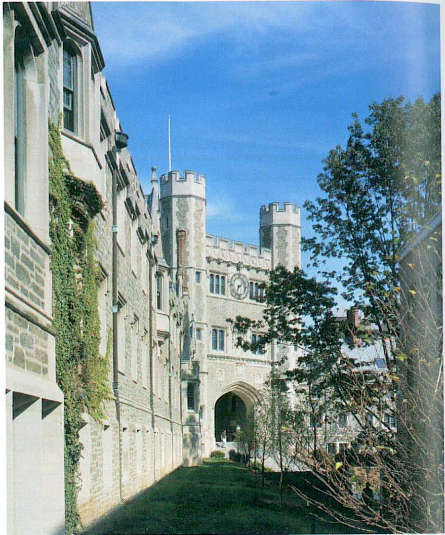
To create more student housing, the existing floor level of the basement was lowered by 18 inches, and new window openings were punched in the south facade to create bright new student rooms. In all, a total of 28 new casement window surrounds were set within tooled limestone surrounds.
