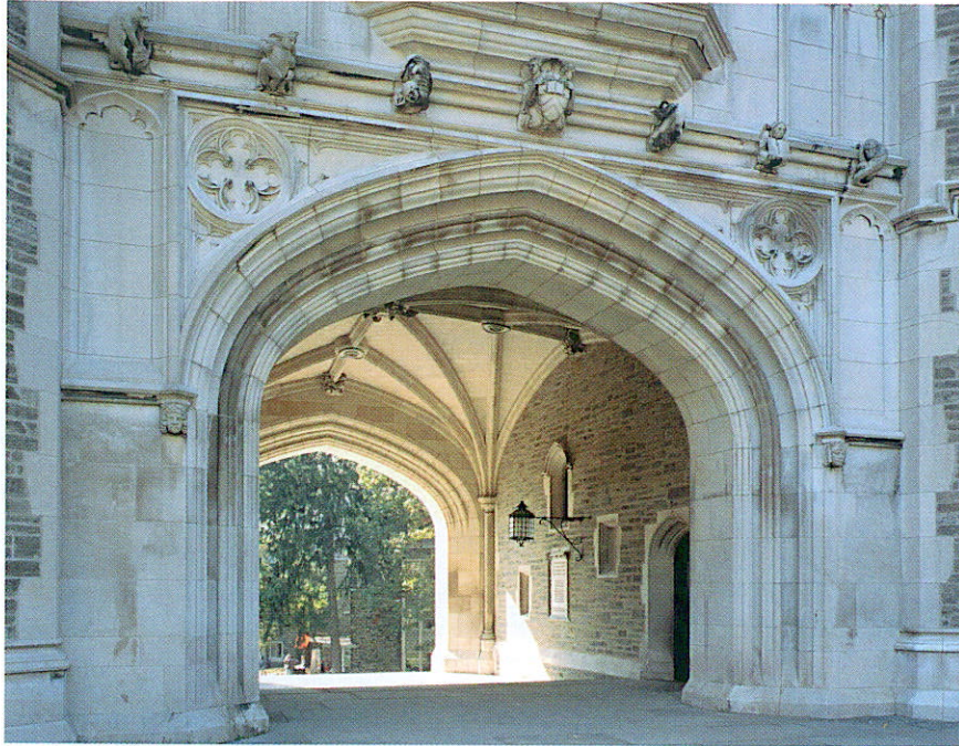
A critical aspect of the project was to ensure that the new stonework would be completely imperceptible from the existing 100-year-old stonework.
