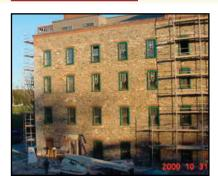
The Mill, White Clay Creek, DE Owner: White Clay Mill Associates Engineer: Landmark Engineering Scope: Restoration of rubble stone facade on Historic mill, Stucco removal, Stone cleaning, repointing. Complete restoration of brick arches at various window locations.
